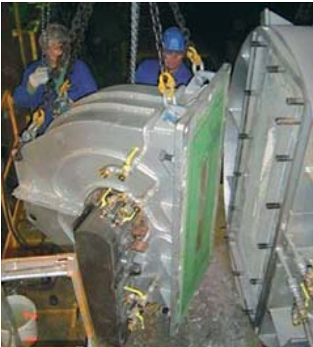
The bottom inductor is flanged into place.
